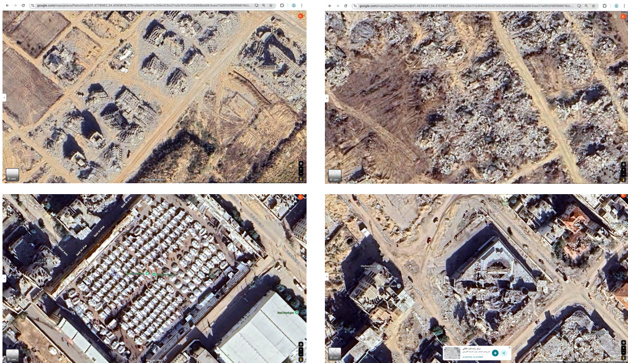
Figure 20 (top and bottom). Destroyed buildings: Google Earth images of destroyed structures in Palestine, 2025. Image by: Google Earth.
